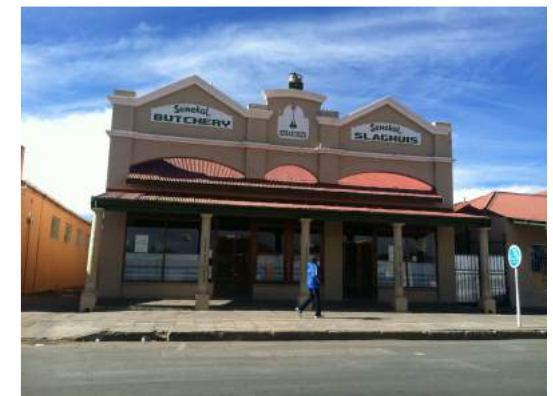
Older (historic) buildings in town
